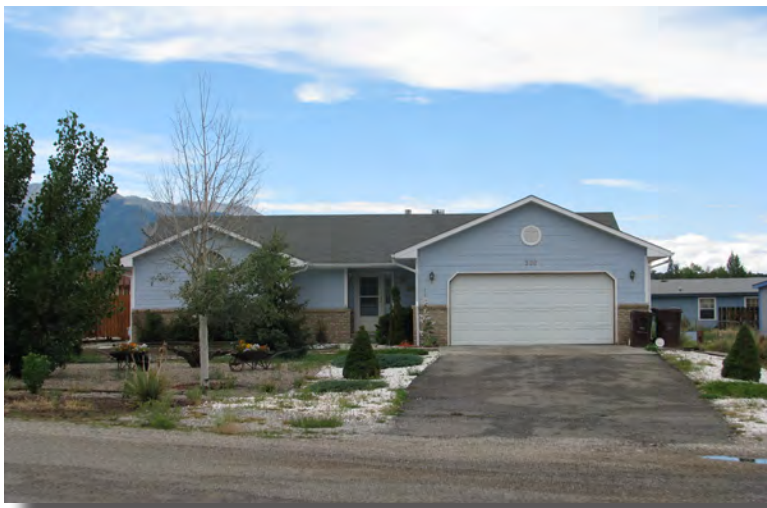
Single Family Dwelling in the Rio POCO neighborhood
