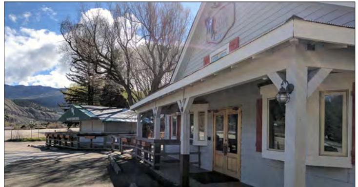
The Wolcott Yacht Club (Wolcott, Colorado) is a business located in a remote location that has achieved success by establishing itself as a unique destination. Riverfront South businesses should consider a similar model in order to find success in the Confluence.
